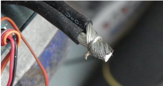
*Fig.5 Initial setup to join two 8 AWG wires, binding wire can be trimmed later*
