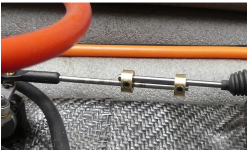
Photograph shows a typical adjustable control rod set up. ©GNP
